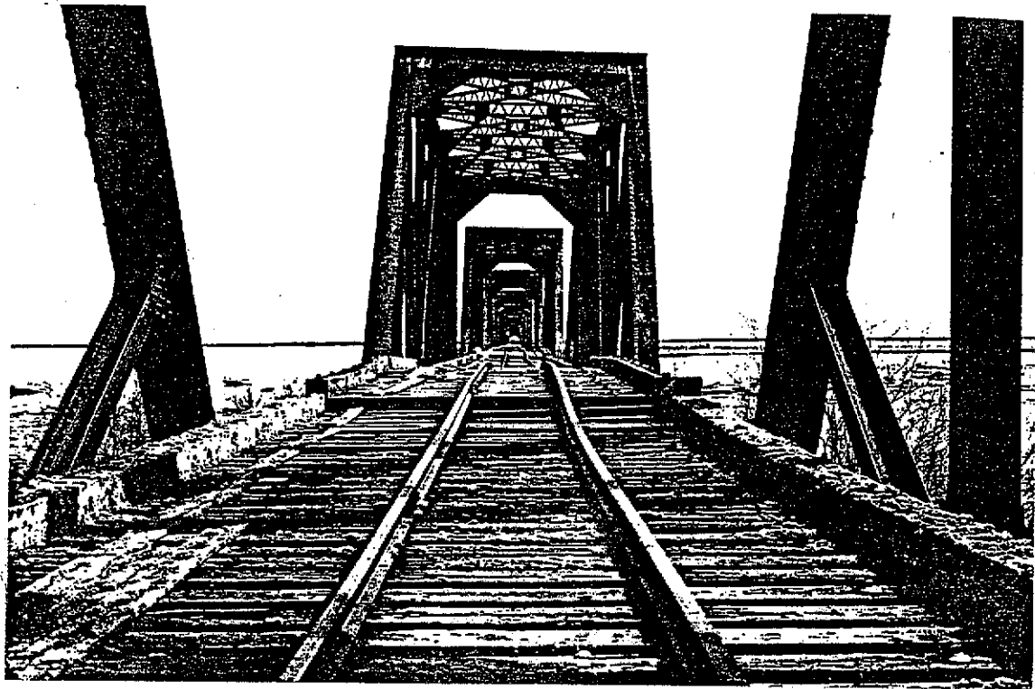
Figure 6: Condition of bridge in 1990, showing the settlement of the truss due to decay of bearing pad. (McLeod report, 1990, Manitoba Culture, Heritage and Recreation)
